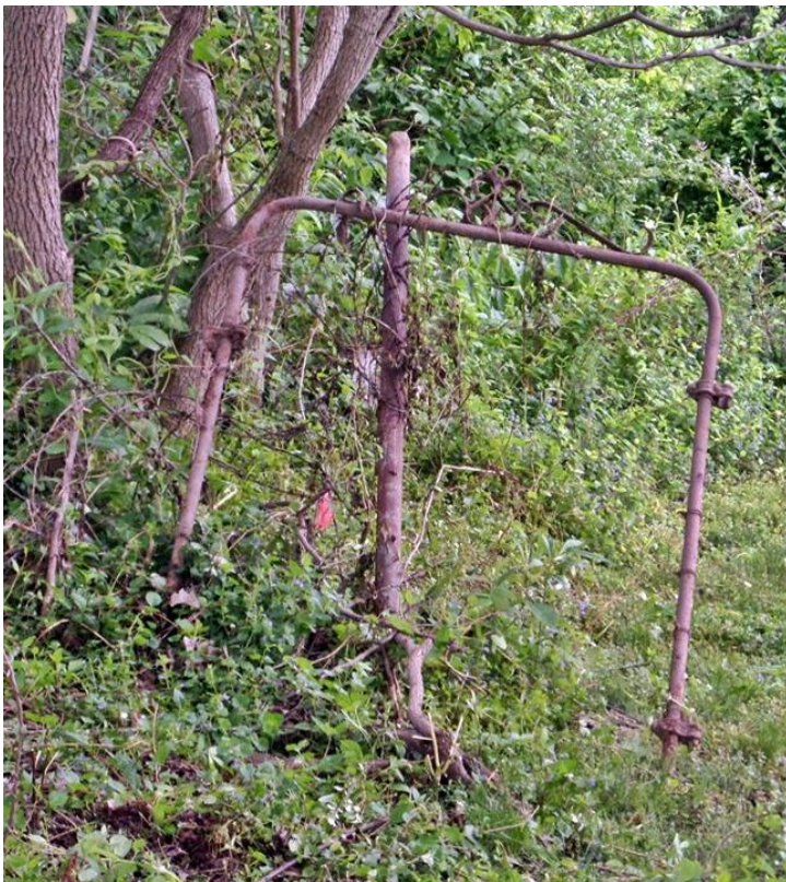
What's left of the old gate. The posts had all rusted off at the ground and the rails were buried in years of plant debris, briars and vines
